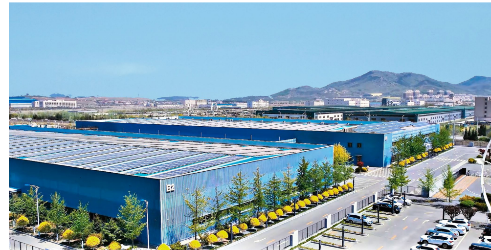
RKP BESS facility producing over 1GW VFB per annum
